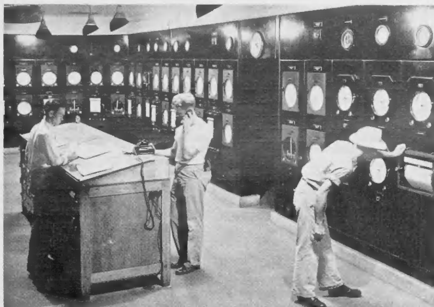
THE CAT Plant control room, left, was a modern installation back in 1944. Many long-service employees probably recall Horace Simmons, shown on the telephone, and the instrumentation, which is large by today's standards. A modern control room, right, has many electronic instruments in addition to pneumatic controls. The console operator merely has to flick a switch to read temperature recordings.
